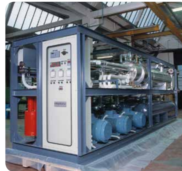
Package units for cascade system, 40 kW capacity at -80°C, condensing with glycol water at -25°C, 3 independent circuits. Refrigeration system for the production of antibiotics.
