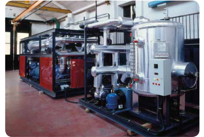
Brine package chilling units down to -75°C cascade system, equipped with pumps and liquid tank. Refrigeration system for the production of antibiotics.
