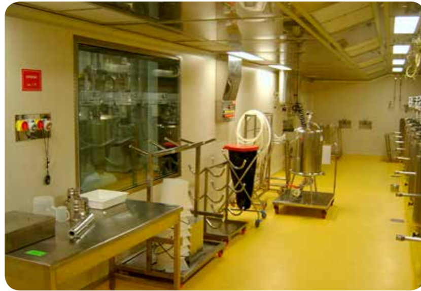
Clean room: cold storage room at -5°C classified in class C.
