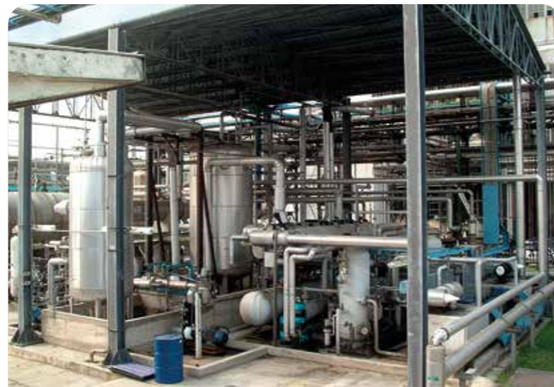
Refrigeration system for the production of antibiotics
